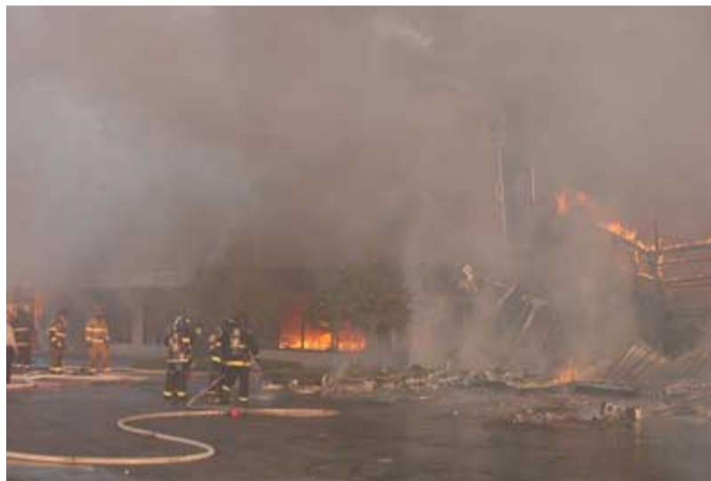
Photo A-4. Time approximately 1951 hours. Front façade beginning to collapse.
