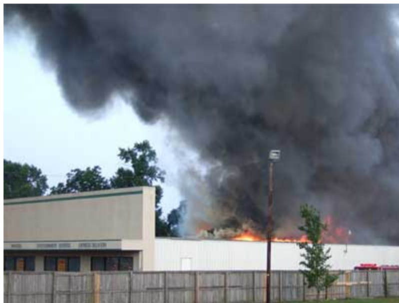
Photo1. Time approximately 1924 hours. Fire is visible over showroom roof. Smoke is dark gray in color and becoming turbulent. The flames may not have been visible from front parking lot or close to the building on the D-side.
