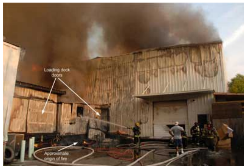
Photo A-2. Time is approximately 1936 hours. Loading dock area approximately 20 minutes after first crews arrived on scene. Note heat damage to metal siding on loading dock and warehouse. (Photo courtesy of Police Department, Bill Murton, photographer.)
