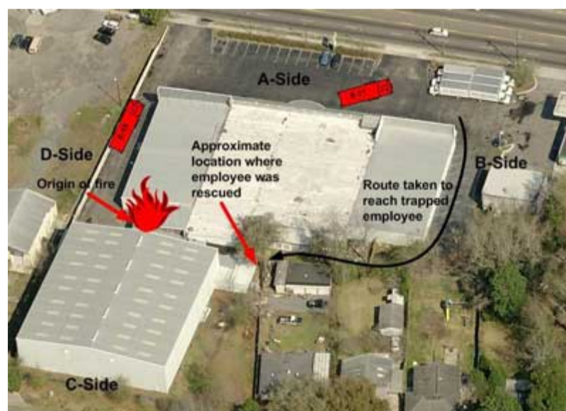
Diagram 3: Note location where mutual aid crew cut through exterior wall to extricate male employee trapped inside the warehouse. From aerial photo taken in 2007. (copyright Pictometry International – used with permission of Pictometry)
