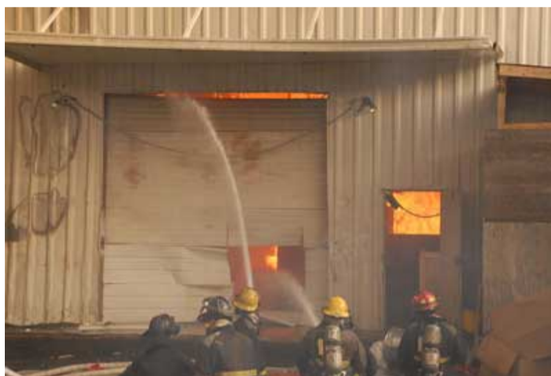
Photo 10. Time approximately 1942 hours. Engine 10 and Engine 12 crews battle fire in warehouse from outside.
